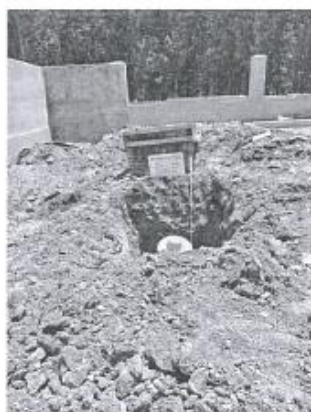
1#危废暂存间北侧
